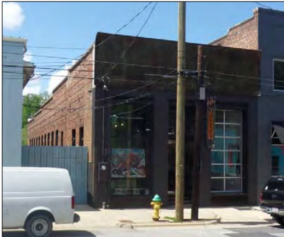
Left: Current view of 349 Depot Street
