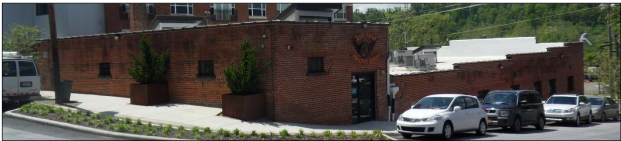
Above: view of 362 Depot Street, facing southwest
