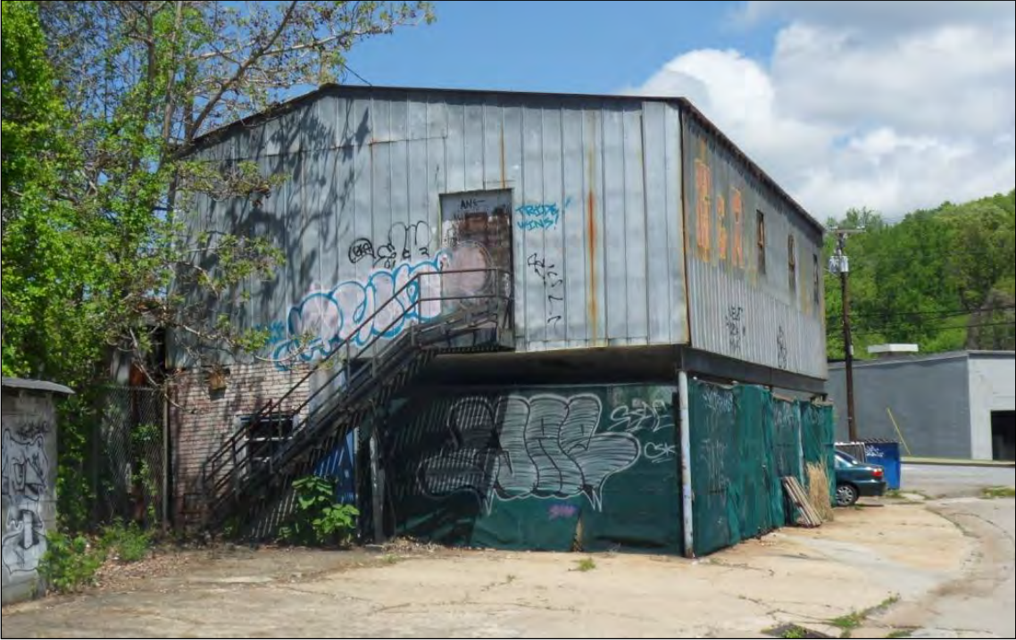
Below, photo shows southern elevation (facing northeast).
