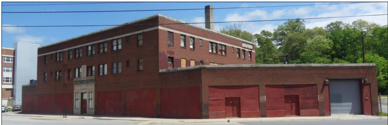
Above: Current view of the Glen Rock Hotel
