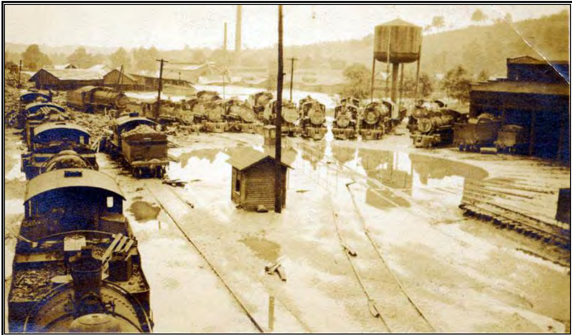
Figure 30 (top). The Southern Railway north of the roundhouse during the Flood of 1916. View to north. Courtesy North Carolina Collection, Pack Memorial Library. Figure 31 (btm). The Southern Railway roundhouse during the Flood of 1916. View to north. Courtesy North Carolina Collection, Pack Memorial Library.
