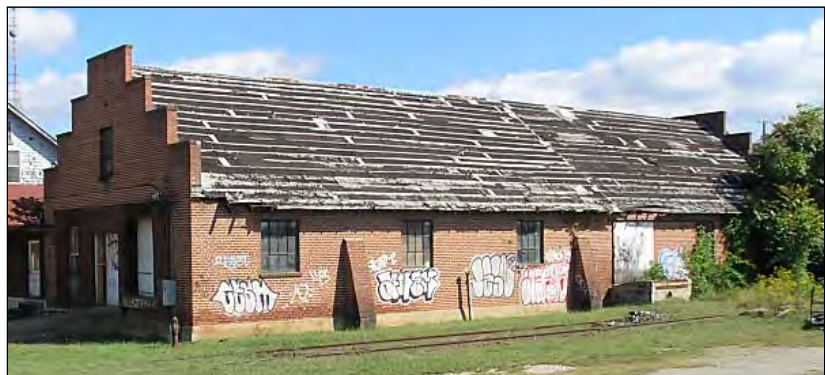
Right: current view of remaining tannery “experimental and chrome building”
