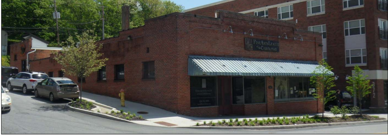
Above: view of 362 Depot Street, facing southeast
