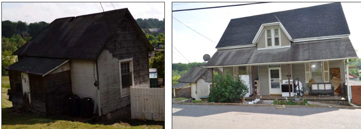
Above: Current view of two buildings at 33 Roberts Street
