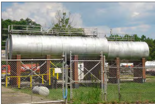
Existing storage tanks, south of buildings
